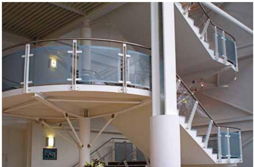
Balustrade infill panels with unperforated margins
