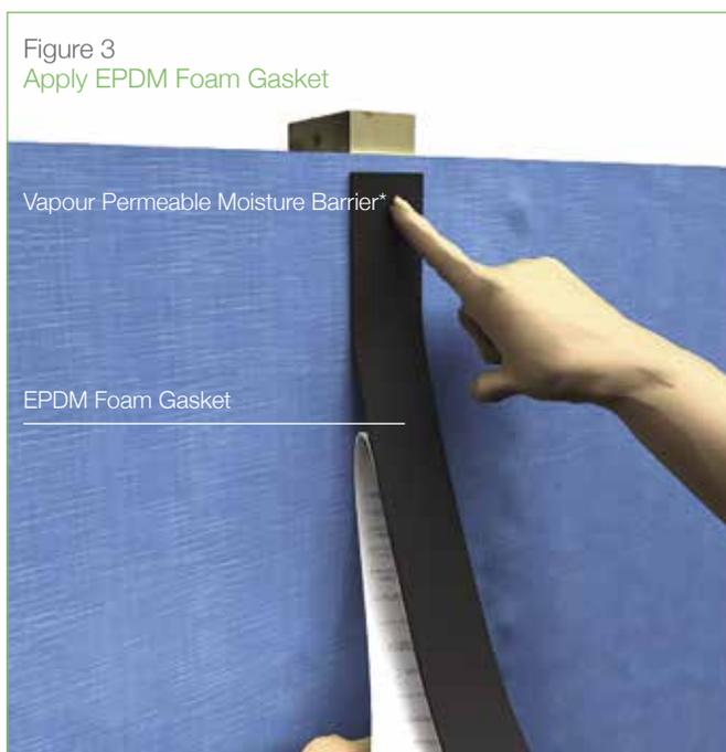
At every vertical joint, fix a continuous strip of EPDM Foam Gasket to the vapour permeable moisture barrier along the stud. This assists to prevent moisture ingress at the sheet joints.
