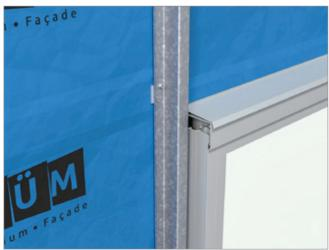
Packers for a plumb substrate and ventilation need to be installed as required prior to the installation of the Stryüm S Batten.
