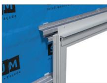
Install the vertical trims for the cladding, at the left and right of the cladding section, at either side of any wall penetrations, and at any corners.
