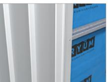
Install the external corner, whilst making sure to cover the screws used to face fix the cladding on the adjoining wall.
