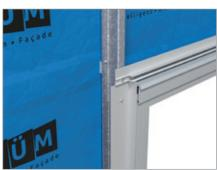
Install the horizontal trims for the cladding, at the top and bottom of the cladding section, above and below any wall penetrations, and at any slab junctions.
