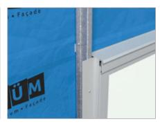
Install the vertical trims for the cladding, at the left and right of the cladding section, at either side of any wall penetrations, and at any corners. When installing down to an adjacent flat surface such as a garden bed or pathway, a minimum of 150mm from the ground is recommended to prevent rain splash back dirtying the façade.
