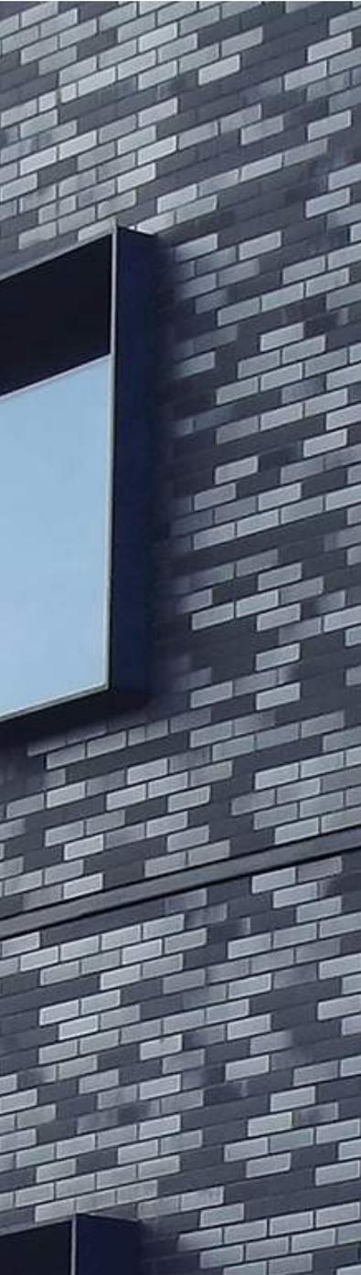
The CORIUM system comprises brick tiles specially manufactured to fix mechanically to an HPS200 galvanised steel backing section. These profiled lengths are mounted in horizontal rows onto a vertical support system and the brick tiles are then clipped in place. The mechanical 'clipping' feature is unique to CORIUM and ensures a high strength façade that enables some adjustment of brick tile position during installation. Mortar is added using a pump system.
