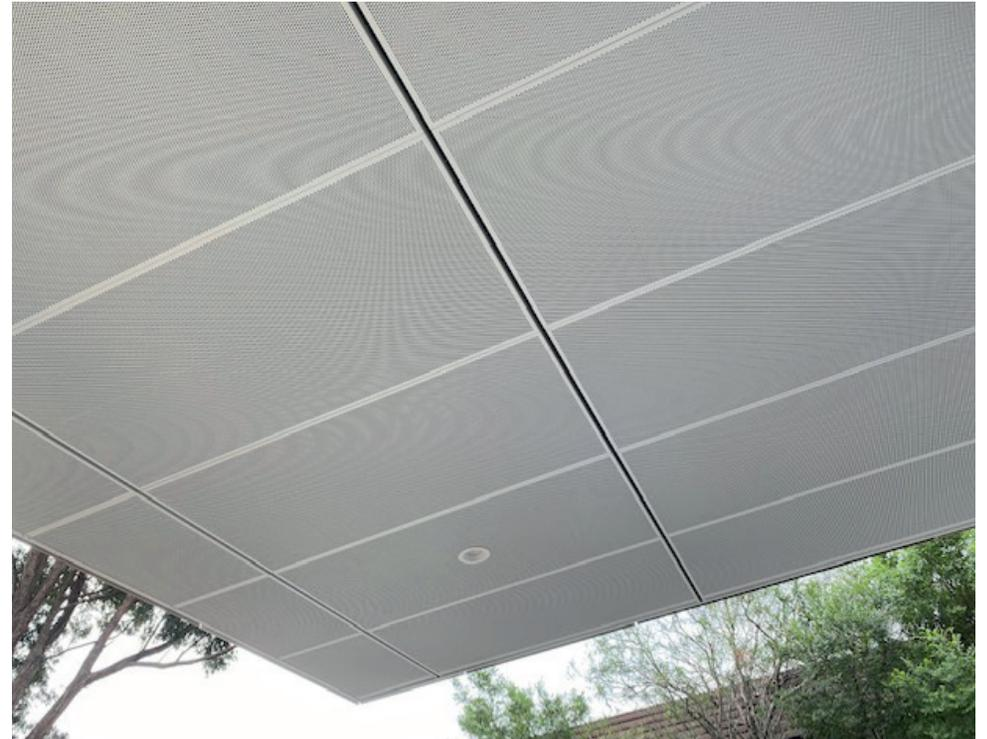
The durlum suspended ceiling system not only met the architect's design brief but allowed it to progress with the building process without delay due to the integration of the durlum system with the Rondo subframe, this resulted in time savings.
